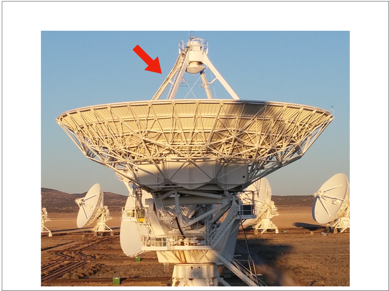
Note the 4 sided support structure! This leads to the square shape of the beams seen on the last slide.
